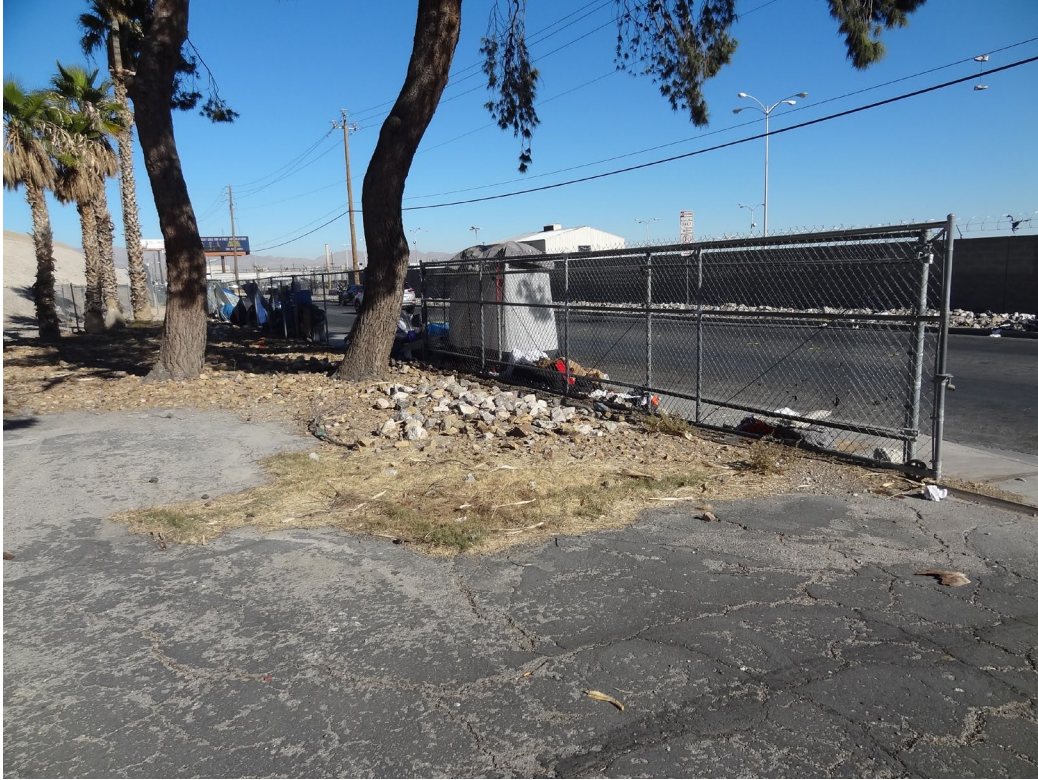
Las Vegas Casual Labor Office Site - Site #9833 Description: Asphalt Parking Lot Replacement Needed.
