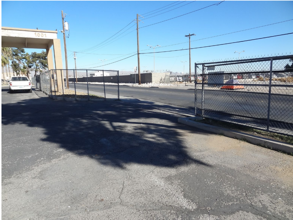
Las Vegas Casual Labor Office Site - Site #9833 Description: Fencing Replacement Needed.
