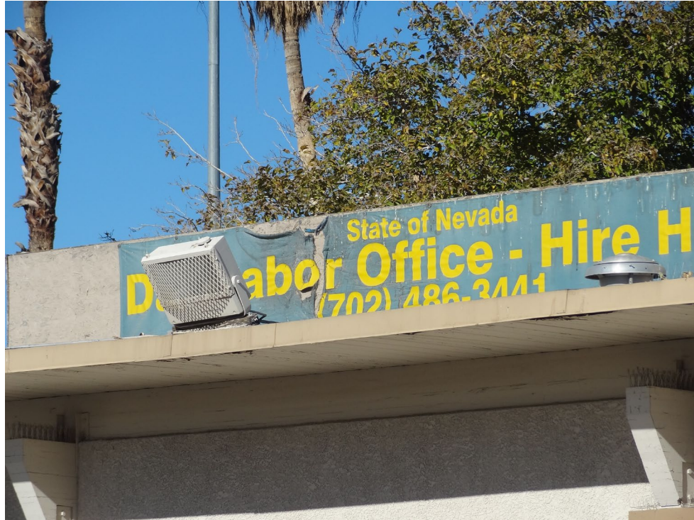
Las Vegas Casual Labor Office - Building #0257 Description: Exterior Lighting Upgrade.
