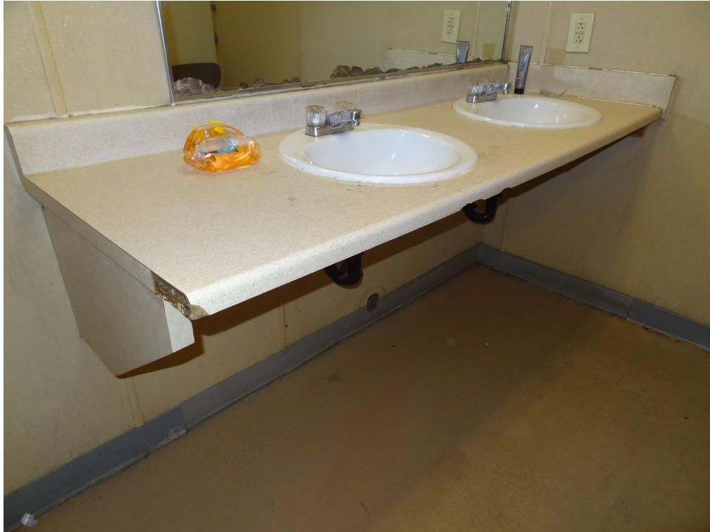
Las Vegas Casual Labor Office - Building #0257 Description: Public Restroom ADA Remodel.
