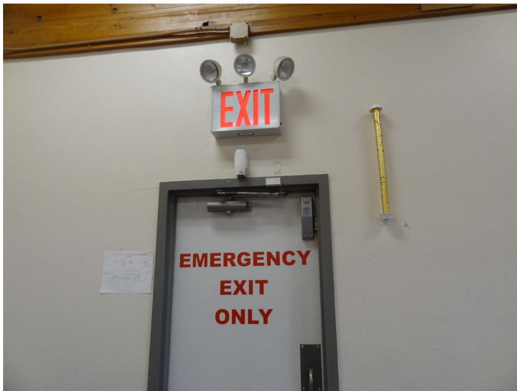
Las Vegas Casual Labor Office - Building #0257 Description: Exit Sign and Egress Lighting Upgrade Needed.
